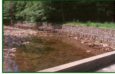
Permanent Gabion in Creek bed
