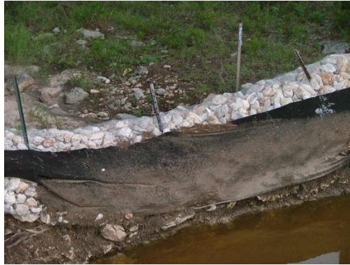
Temporary Gabion and Silt Fence
