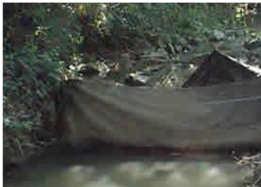
Silt Fence in Creek Bed
